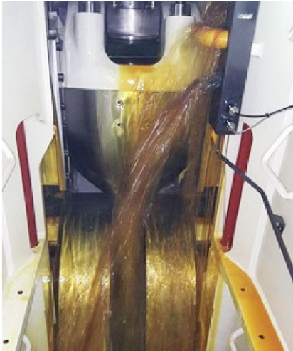
Inspection of Oil Flow
